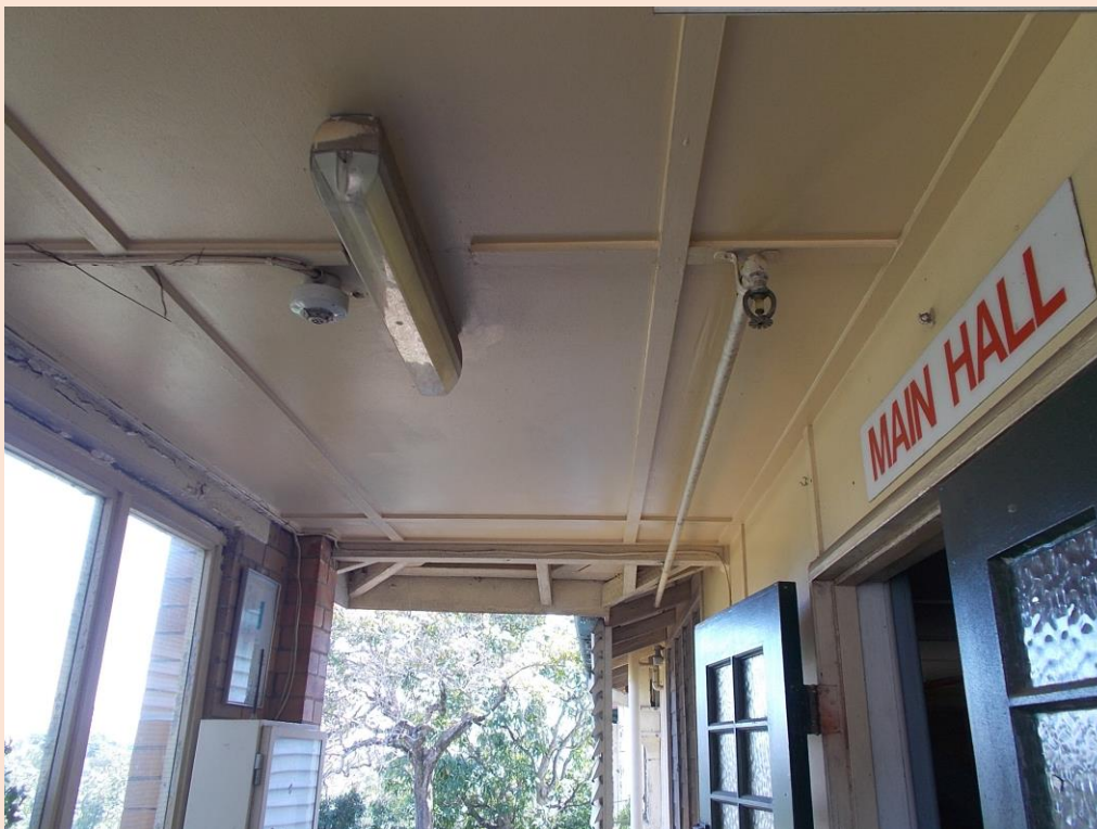
Image 2: Front verandah entrance ceiling is lined in asbestos cement sheet.
