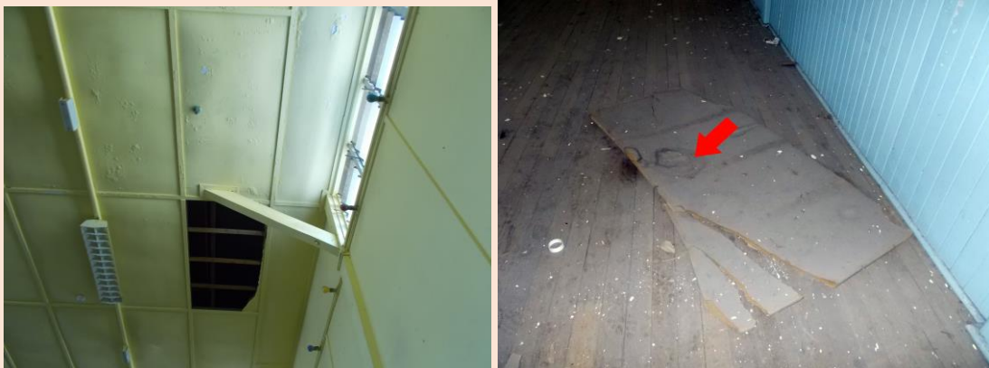
Image 17: It should be expected that upper structural supports and beams will be contaminated with asbestos that has gradually released over decades from the former asbestos cement roof cladding. Even a wooden ceiling panel which had fallen to the floor and been sitting there for a number of years was found to be contaminated on its top surface (sample DV – 02)
