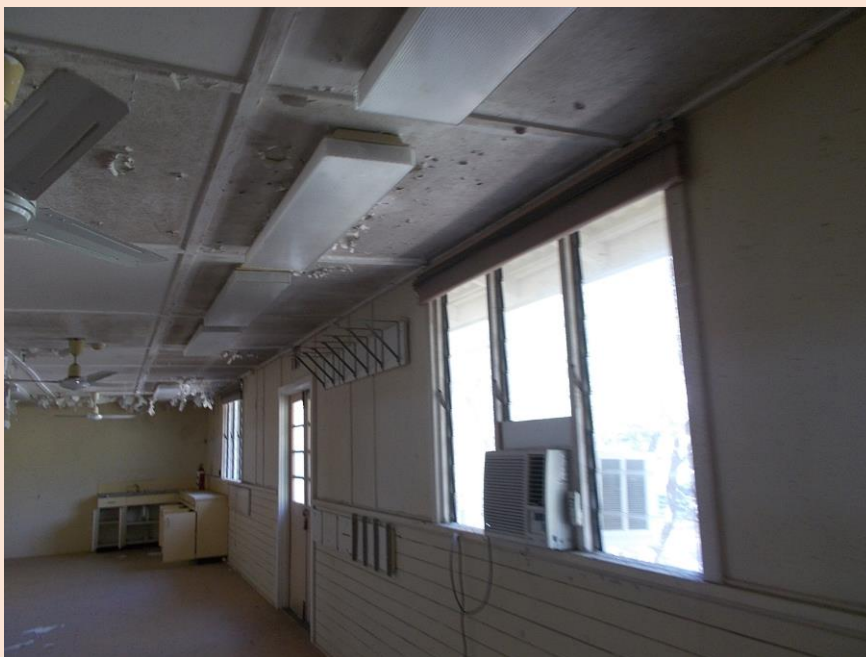
Image 12: The walls and ceilings to all the lower ceiling areas on both sides and rear of the Hall itself including the two Units are lined in asbestos cement sheeting.
