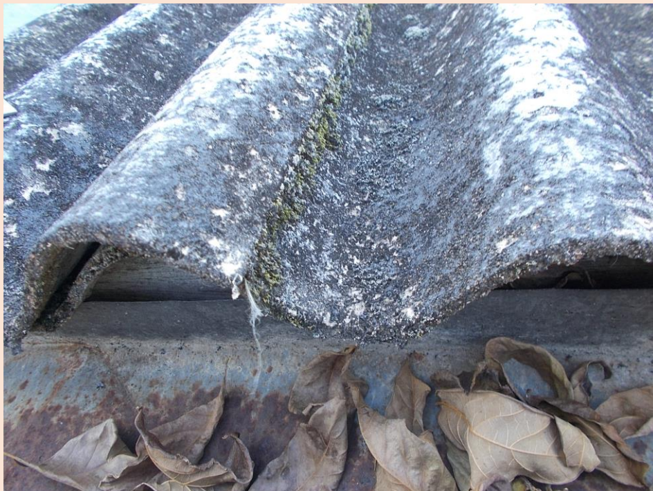
Image 6: Some of the sealant still remains where it's not as exposed to the weather but as can be seen the rest of the roof cladding is in poor condition.
