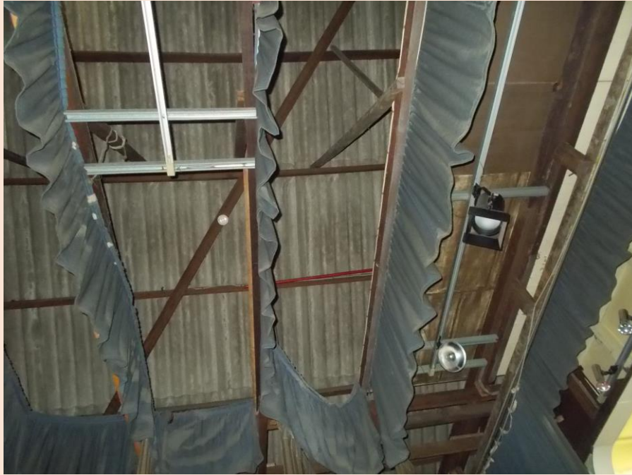
Image 16: Open ceiling space to the corrugated asbestos cement roof behind the Stage
