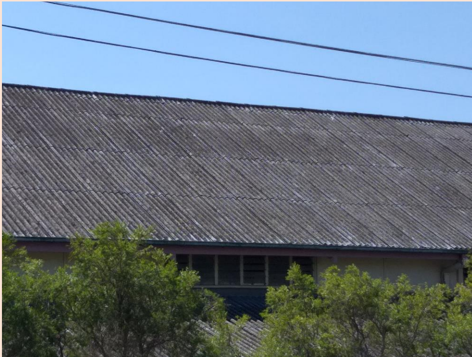
Image 4: The steep pitch means that asbestos released from the deteriorating roof washes down into the gutter and over it.
