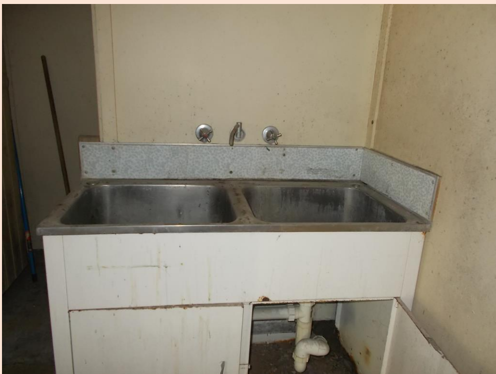
Image 19: The sink backing panels are constructed of laminated asbestos cement sheeting.
