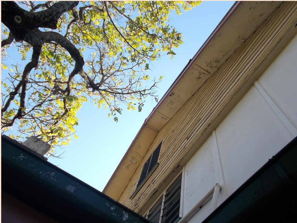
Image 10: The external upper eaves (under the end pitched rooves) are lined in asbestos cement sheeting.
