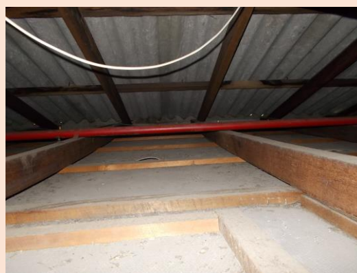
Image 15: Former Kitchen Lunchroom ceiling space this year (2019) where a sample (DV – 01) was taken this was positive for asbestos.
