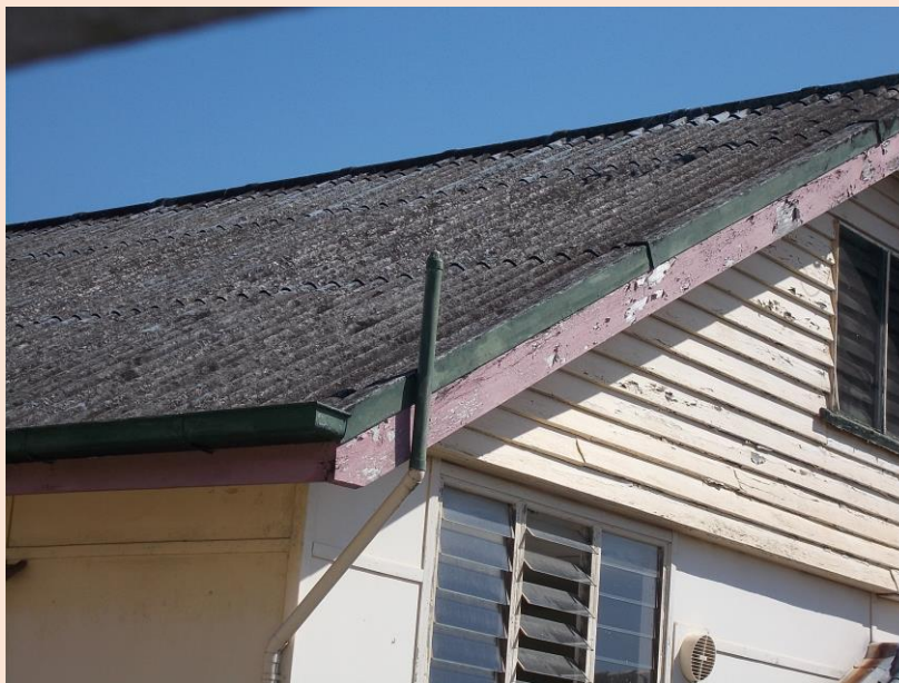
Image 20: The roof cladding is corrugated asbestos cement sheeting.
