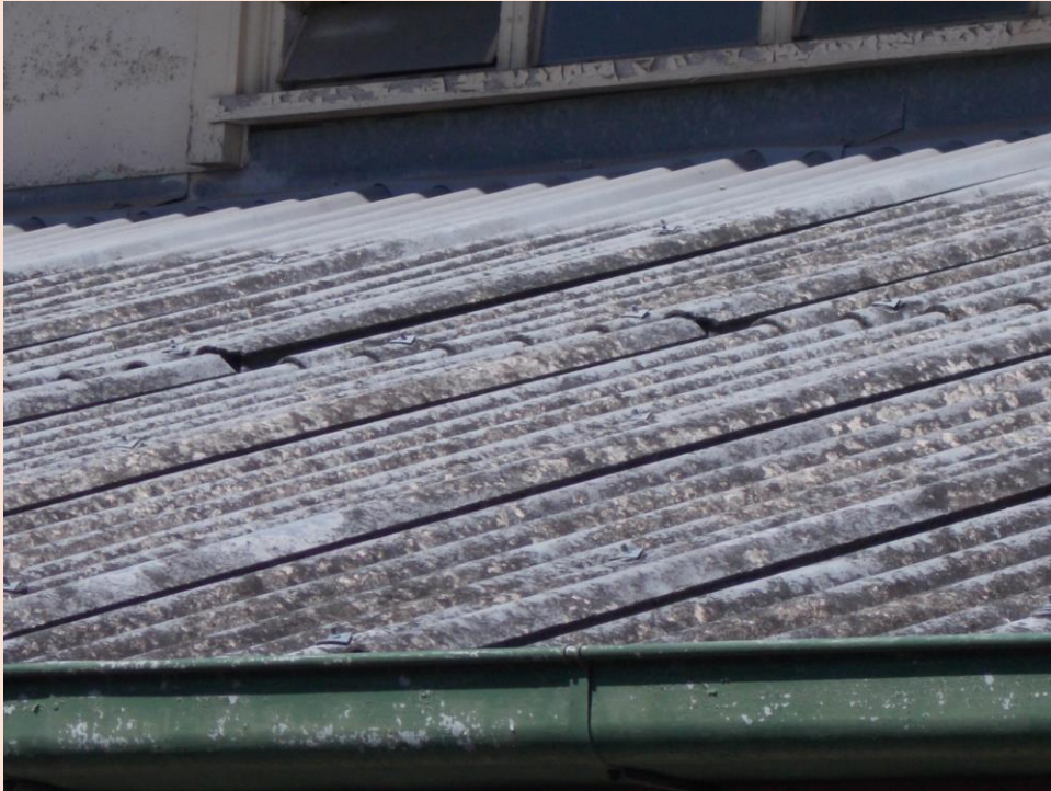
Image 6: Some of the sealant still remains where it's not as exposed to the weather but as can be seen the rest of the roof cladding is in poor condition.
