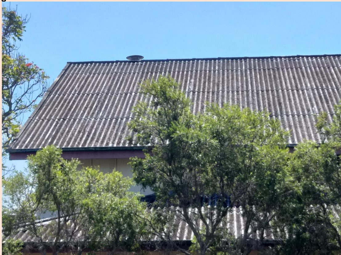
Image 3: Steep pitch corrugated asbestos cement roof cladding.
