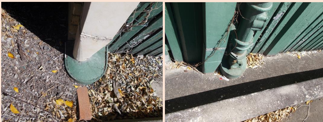
Image 1: External drain surrounds are asbestos cement.
