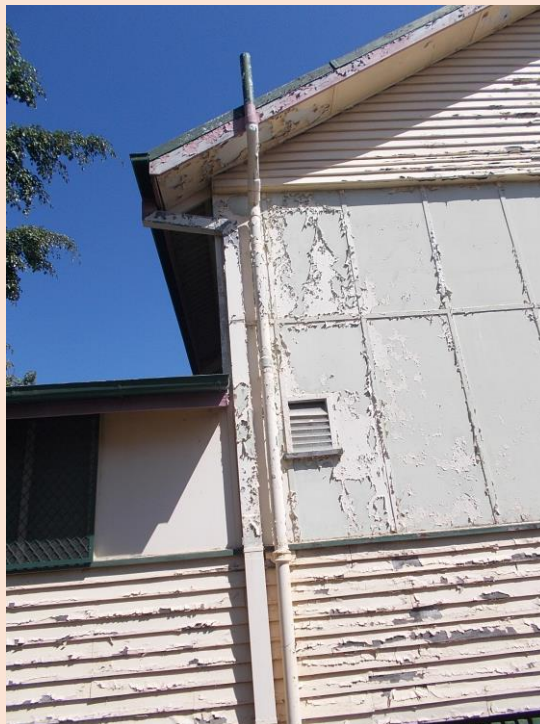
Image 11: The sewerage vent pipe extending up from the ground at the rear of the Main Hall Building has an asbestos cement pipe upper section.
