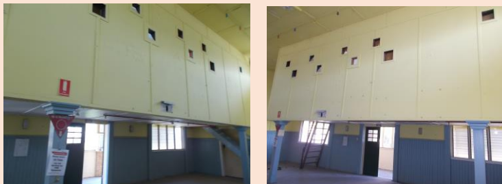
Image 13: Projector Room: Outer wall and underside ceiling lined in asbestos cement sheeting.
