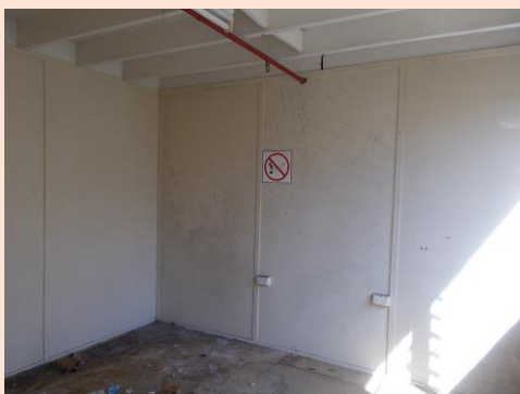
Image 18: Downstairs rooms showing the asbestos cement sheet used for the walls.
