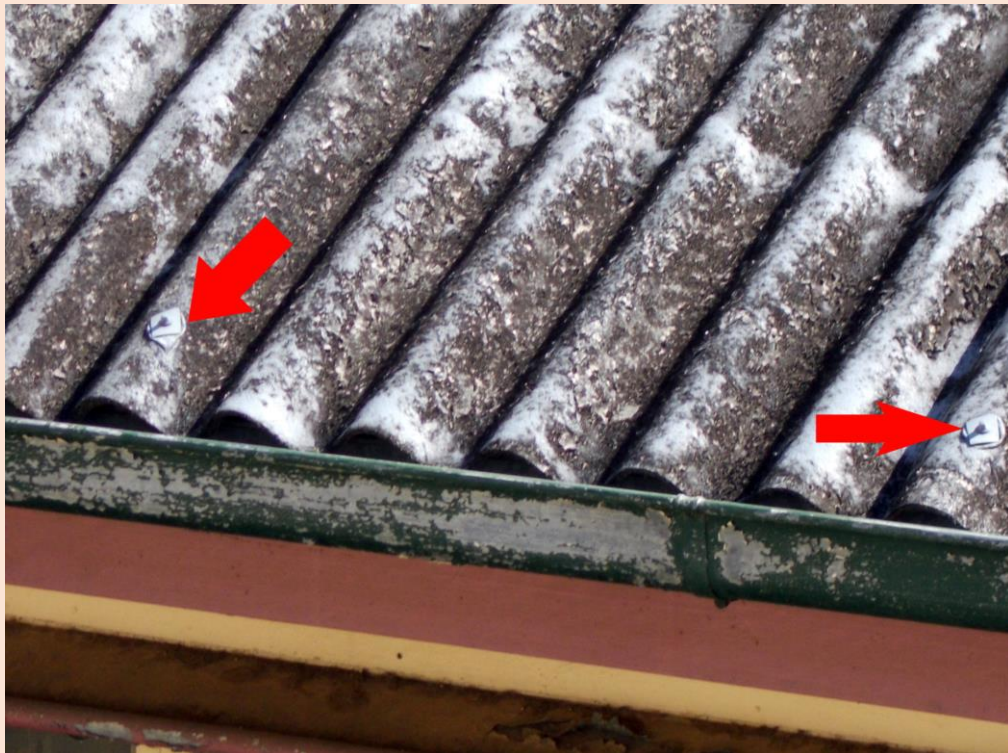
Image 23: The black sealant (painted grey) used to waterproof around the roofing nails contains asbestos.
