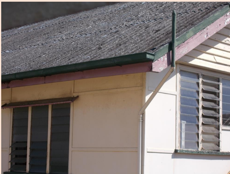
Image 24: The main walls to the outside of the building are clad in asbestos cement sheeting.
