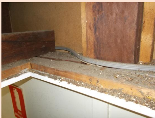
Image 15: Former Kitchen Lunchroom ceiling space this year (2019) where a sample (DV – 01) was taken this was positive for asbestos.
