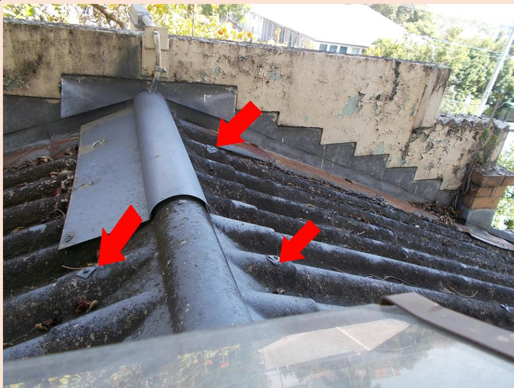
Image 8: The black sealant (painted grey) used to waterproof around the roofing nails contains asbestos.
