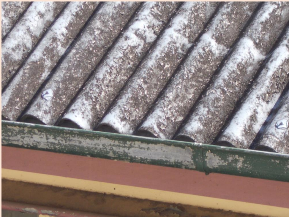
Image 21: Lower rear area of corrugated asbestos cement sheet roof cladding
