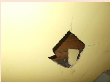
Image 14: Damaged wall panel on the West Staircase.
