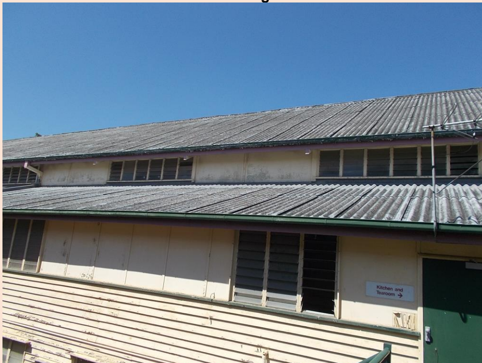
Image 4: The steep pitch means that asbestos released from the deteriorating roof washes down into the gutter and over it.
