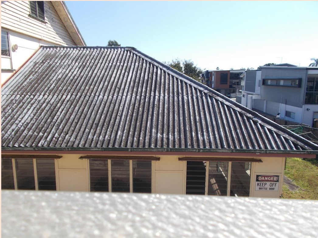
Image 21: Lower rear area of corrugated asbestos cement sheet roof cladding
