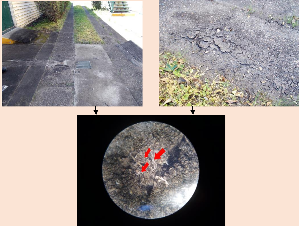
Image 29: Flow chart Illustrating Roof Cladding Breakdown and bottom -Asbestos fibre bundles visible in sample DV - 13 from the area between the buildings.
