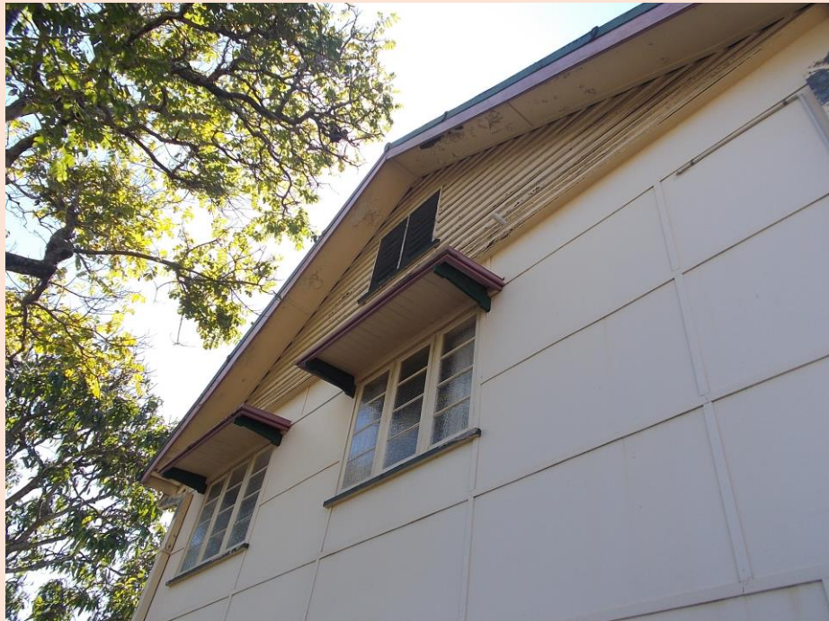
Image 25: The external upper eaves (under the end pitched rooves) are lined in asbestos cement sheeting.
