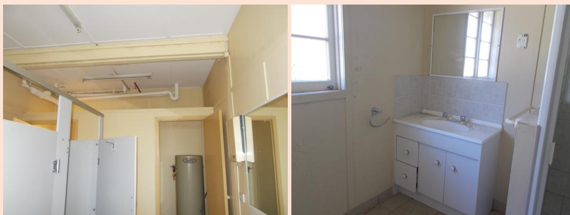
Image 26: Examples of the mix of asbestos cement sheeting, non asbestos cement sheet, wood and plaster panels in the Ablution Areas.
