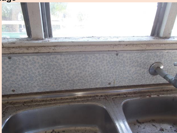
Image 28: The sink backing panels are constructed of laminated asbestos cement sheeting.
