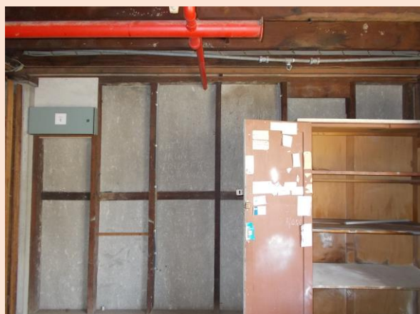
Image 18: Downstairs rooms showing the asbestos cement sheet used for the walls.
