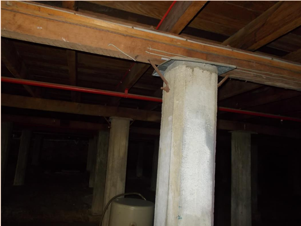
Image 35: Stump Packing Beneath Building: Asbestos cement sheet pieces where commonly used for stump and floor support level packing.
