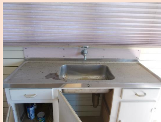
Image 28: The sink backing panels are constructed of laminated asbestos cement sheeting.
