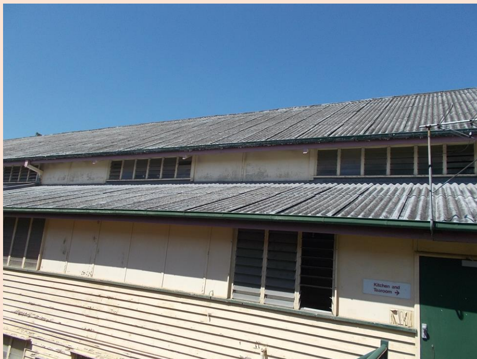
Image 9: Asbestos cement wall cladding around the perimeter of the building.
